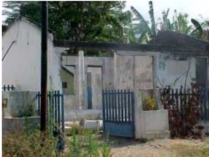
GLENO TRANSMISSION RACK, SERVICE COMPLEX,
