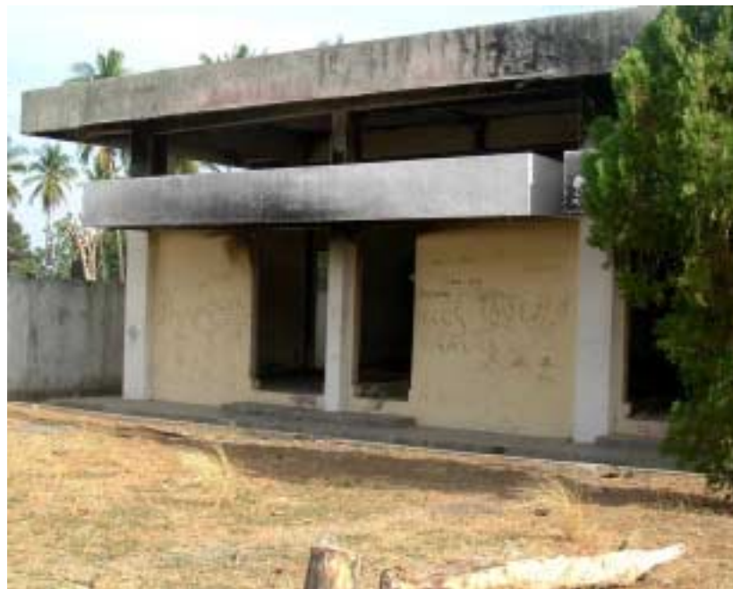
OCUSSI EXCHANGE BUILDING
