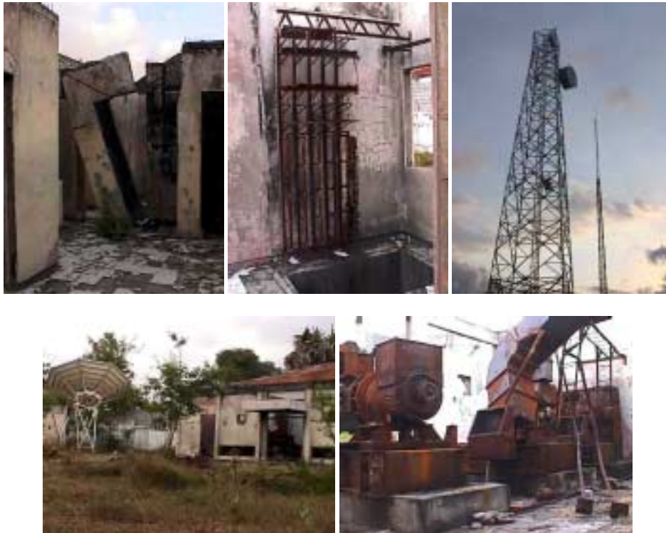
Suai exchange building, MDF room, radio tower, satellite antenna and generator room
