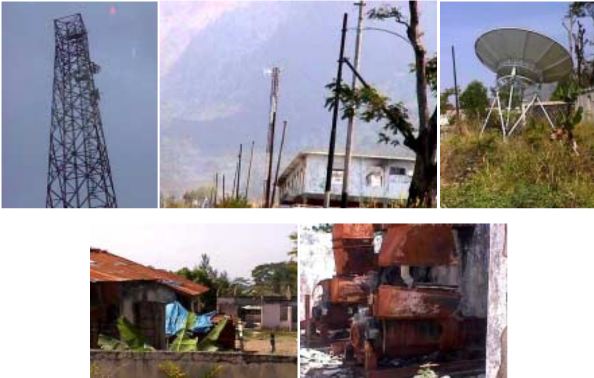
AINARO TOWER, OSP POLES, SATELLITE ANTENNA, SERVICE HOUSES AND GENERATOR HOUSE
